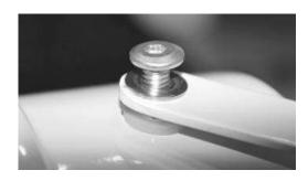
Detail of the mounting of the bracket with bolt, washer and silicon washer.
